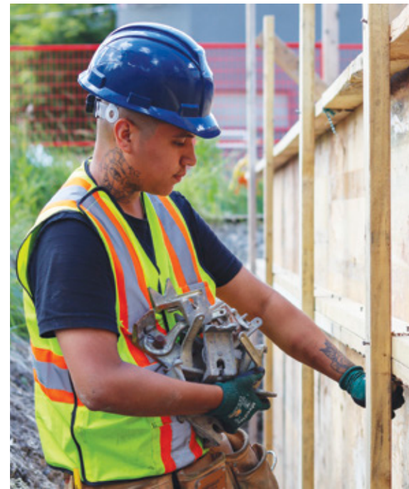
Construction work placement, Purpose Construction
